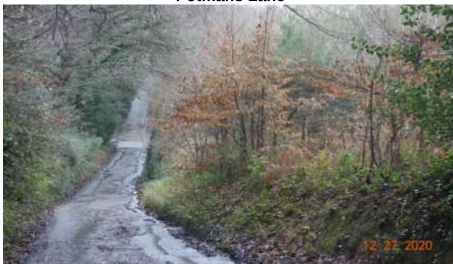
Spratts Lane – liable to flooding across the road (as here) 27 December 2020
