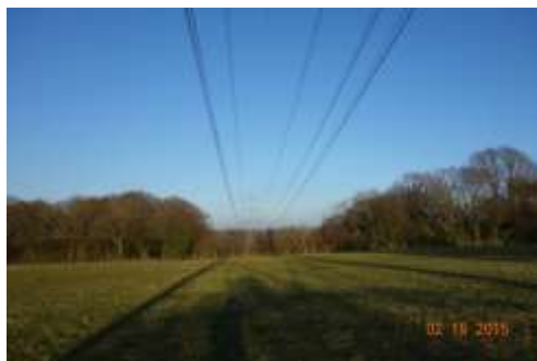
A wayleaf cut through Wayfield Shaw, looking east
